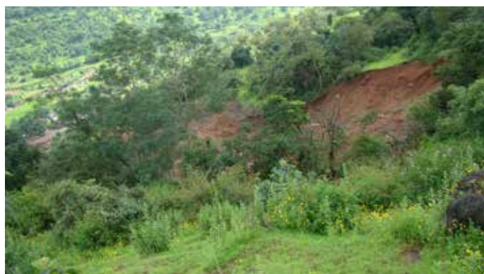
Wide view of main scarp and crown
